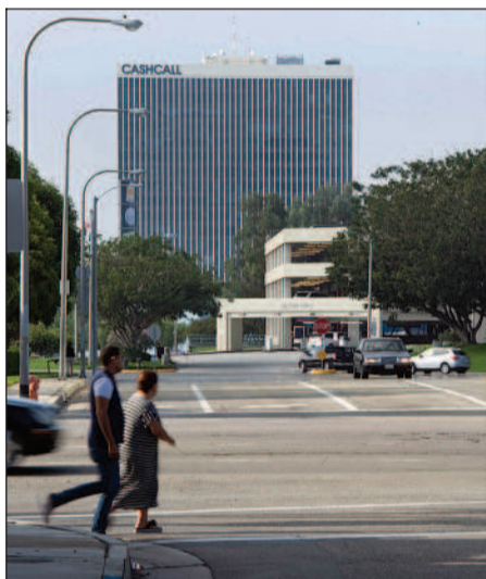
JOSHUA SUDOCK, STAFF PHOTOGRAPHER CashCall headquarters in Orange. Lenders like CashCall can charge any interest rate for loans of $2,500 or over.
